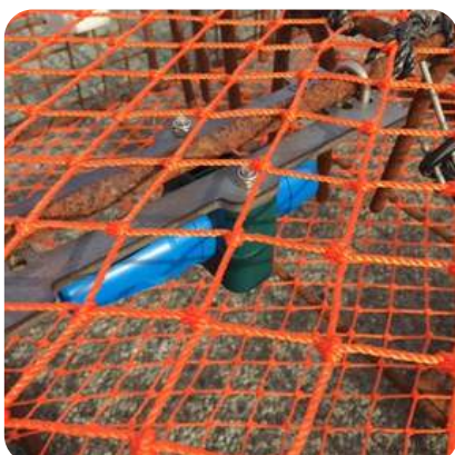
Mounting Plate #2 with Stauff Clamp
